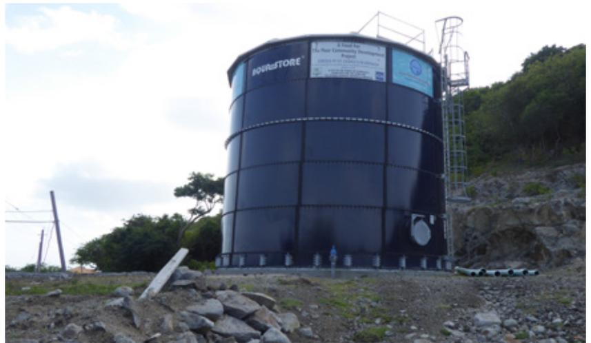
**The storage tank at Laca Pierre is on a hill, allowing gravity-feed distribution of water to local communities.**
