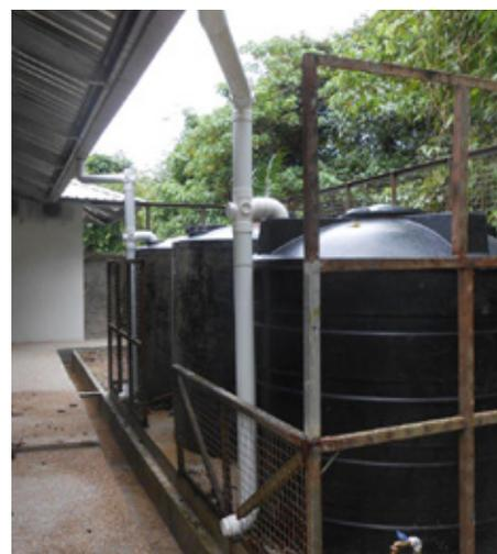
Example of an installed First-Flush Diverter, CARICOM & GWP
